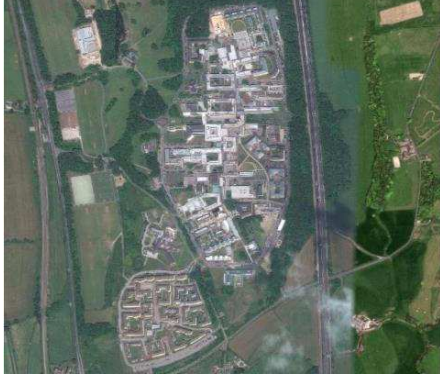
(a) Google Earth view of Lancaster University
